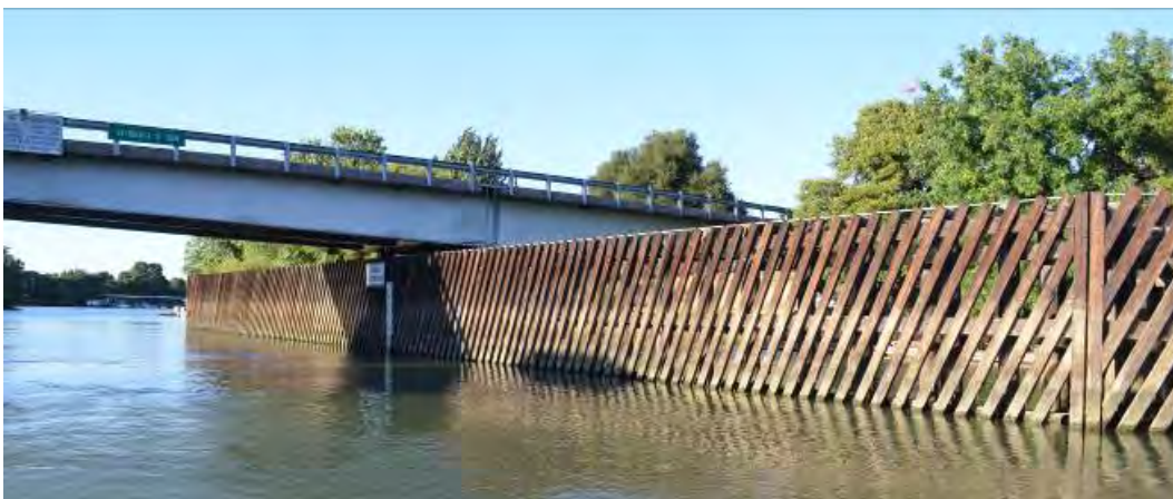
B. Looking north from the main channel.
