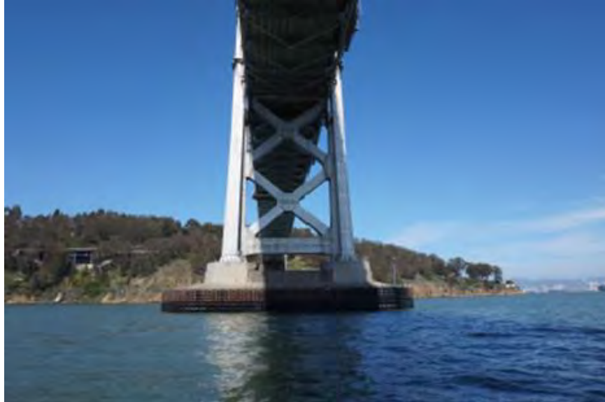
Figure 77. Photo. Pier W6 viewed from the west.
