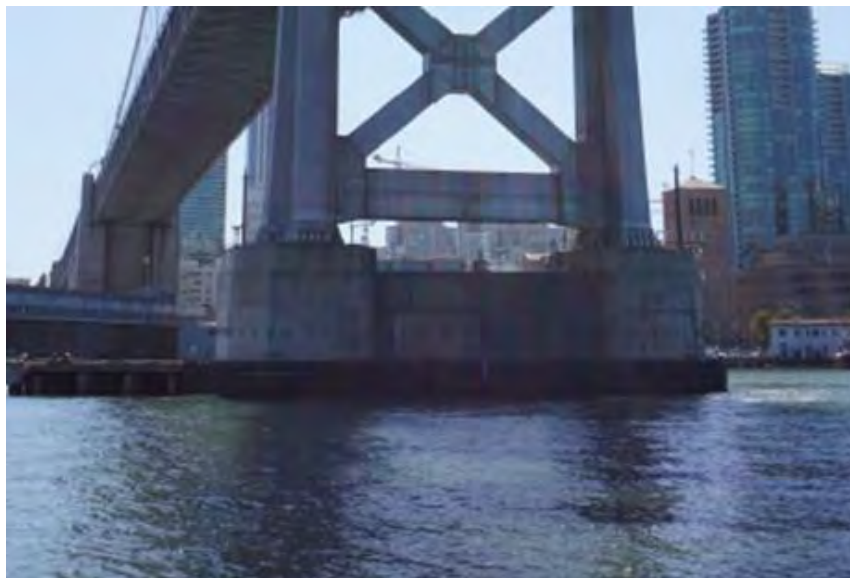
Figure 76. Photo. Pier W2 viewed from the east.
