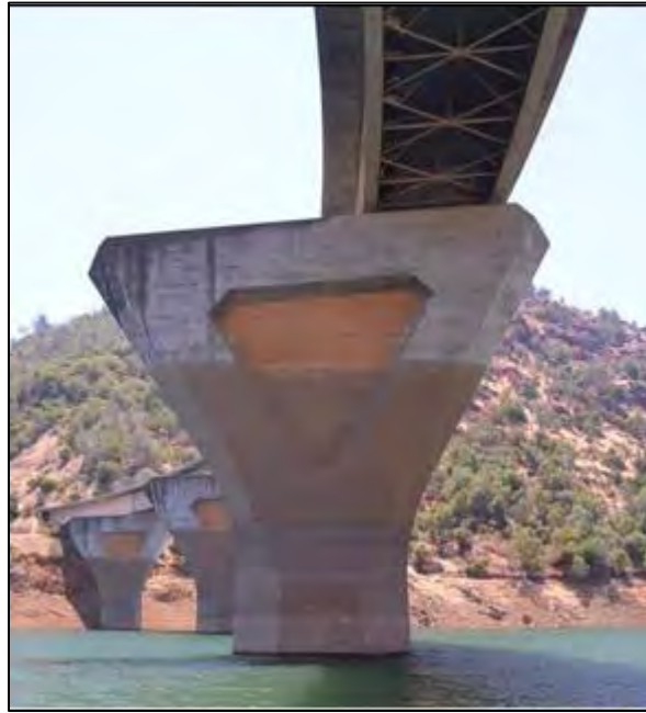
Figure 38. Photo. Northwest face of bent 4.
