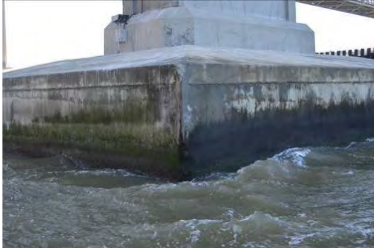
Figure 62. Photo. Tower 3 pile cap close-up.
