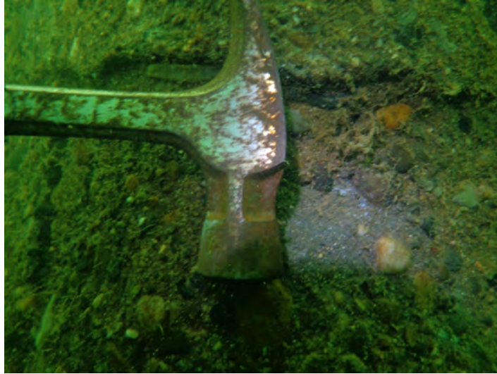
Figure 50. Photo. Typical cold joint after cleaning.
