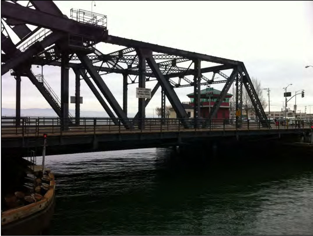
Figure 71. Photo. Third Street Bridge.
