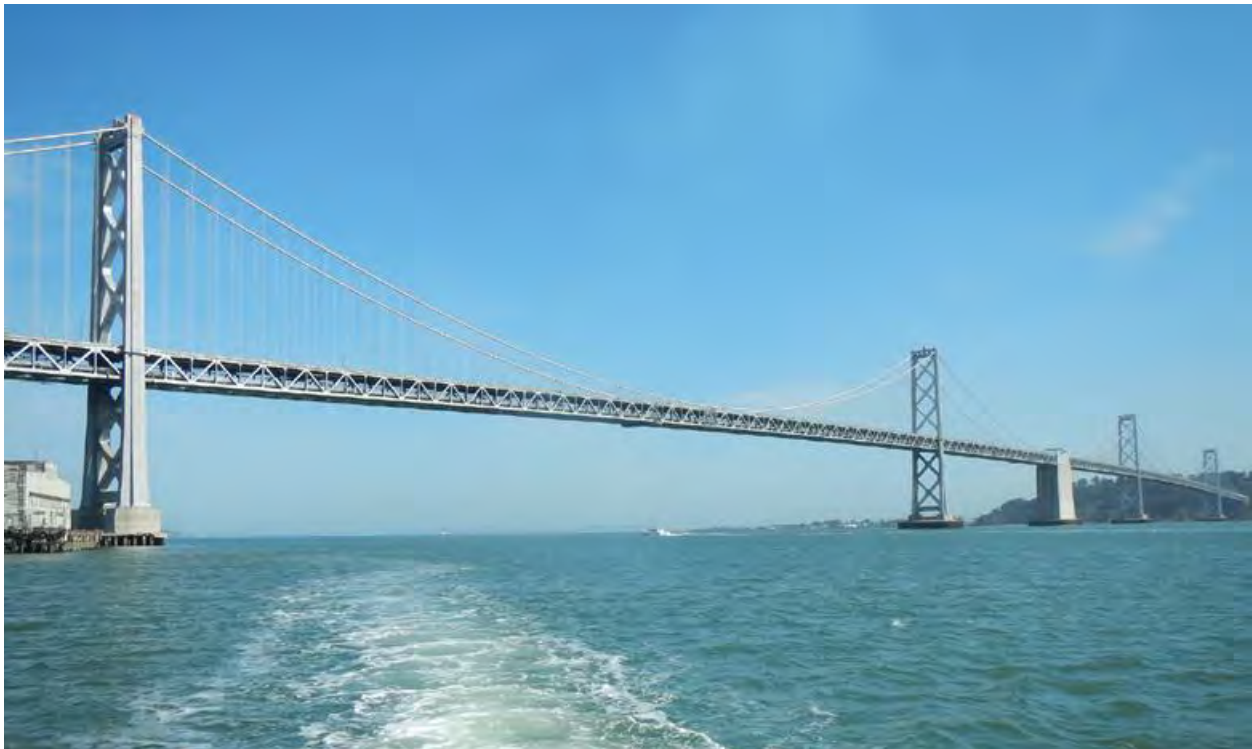
Figure 70. Photo. SF-OBB viewed from the south.
