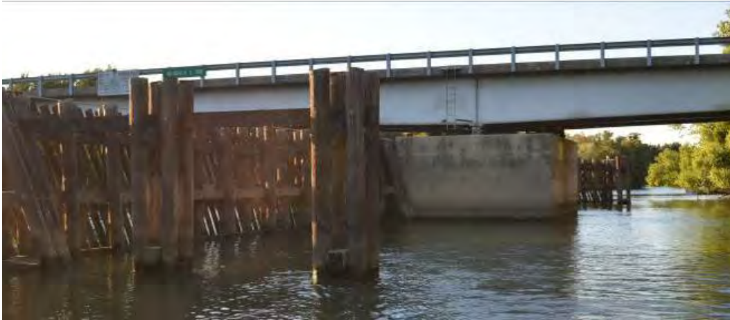
A. Looking north behind the timber fender.
