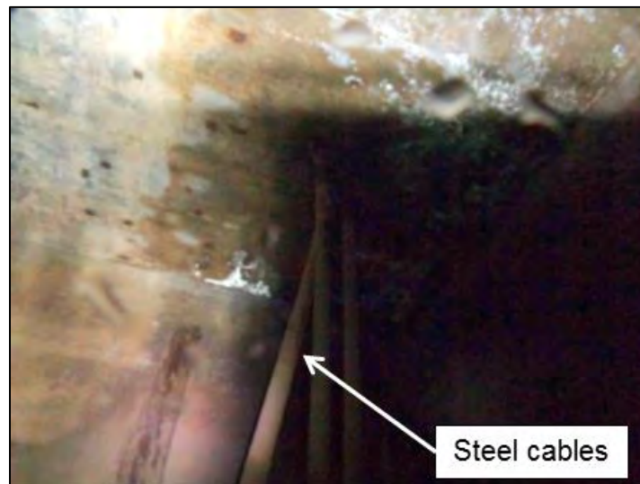
Figure 37. Photo. Above water view of steel cables.
