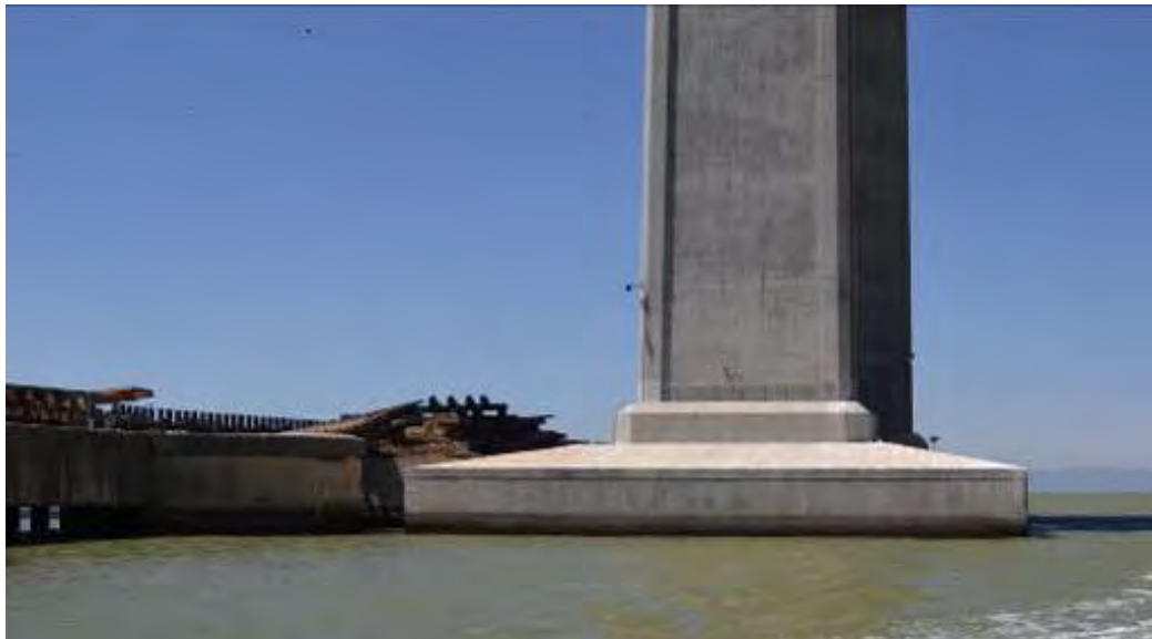
Figure 61. Photo. Tower 3 pile cap.
